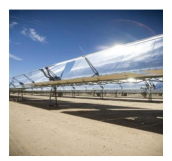
A field of parabolic trough solar collectors
